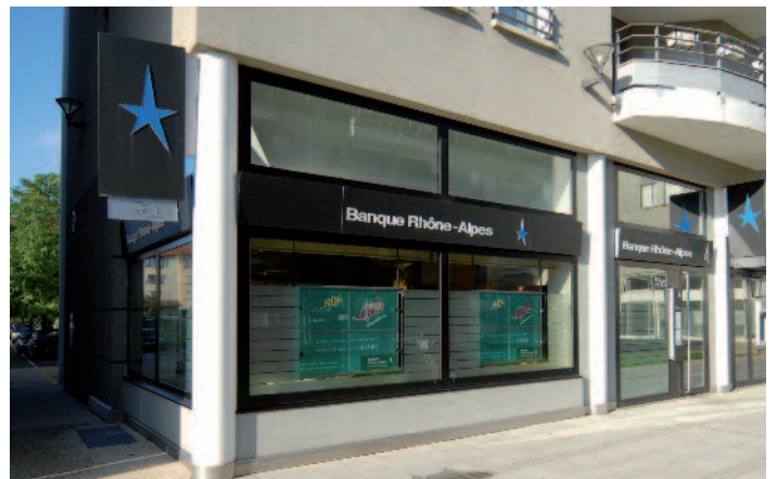
Façade agence Pont-de-Claix / 2006
